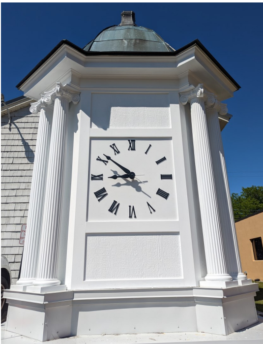
The restored clock tower patiently waited for installation in the Village parking lot.
